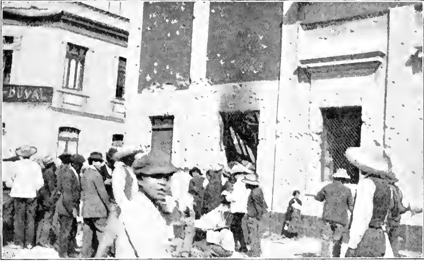
THE WALLS OF THE NUEVA ERA OFFICE AFTER THE BOMBARDMENT.
